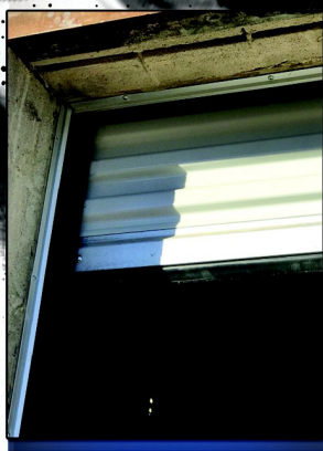
INSTALLS W/ SELF TAP SCREWS
